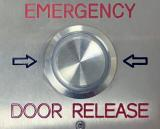
PRESSING THE EMERGENCY BUTTON MOMENTARILY (Press & Release) acts as a power OFF / ON to the EM24EX (Fail Safe Timer Relay) which activates the hold unlocked release feature of the electrical locking for the preset duration period.
